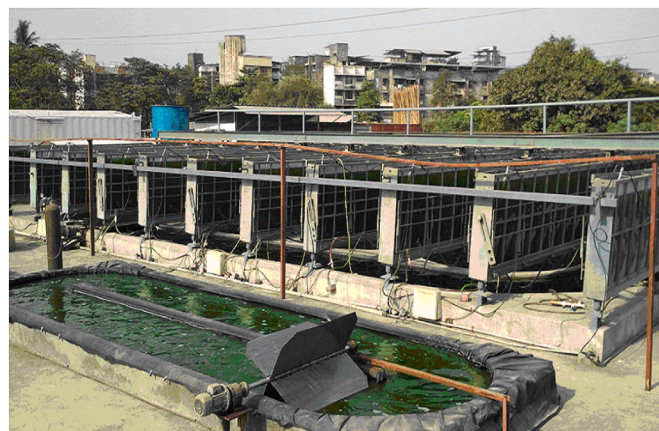
Fig. 7. Sunlight distribution-based open algal growth system (220 sq. m/100,000 L) with a raceway pond inoculum system (6000 L) at The Energy and Resources Institute, Navi Mumbai, India [121].
