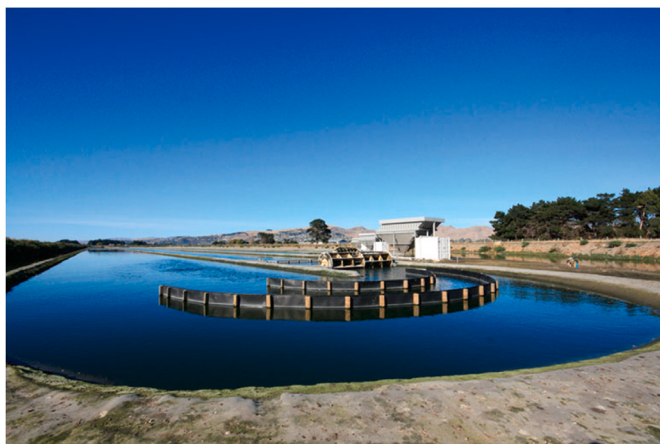
Fig. 6. A large-scale algal raceway pond (1.25 ha) in Christchurch, New Zealand [149].
