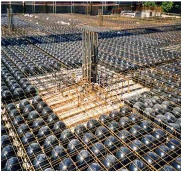
Fig. 1.2. Used In Construction.
